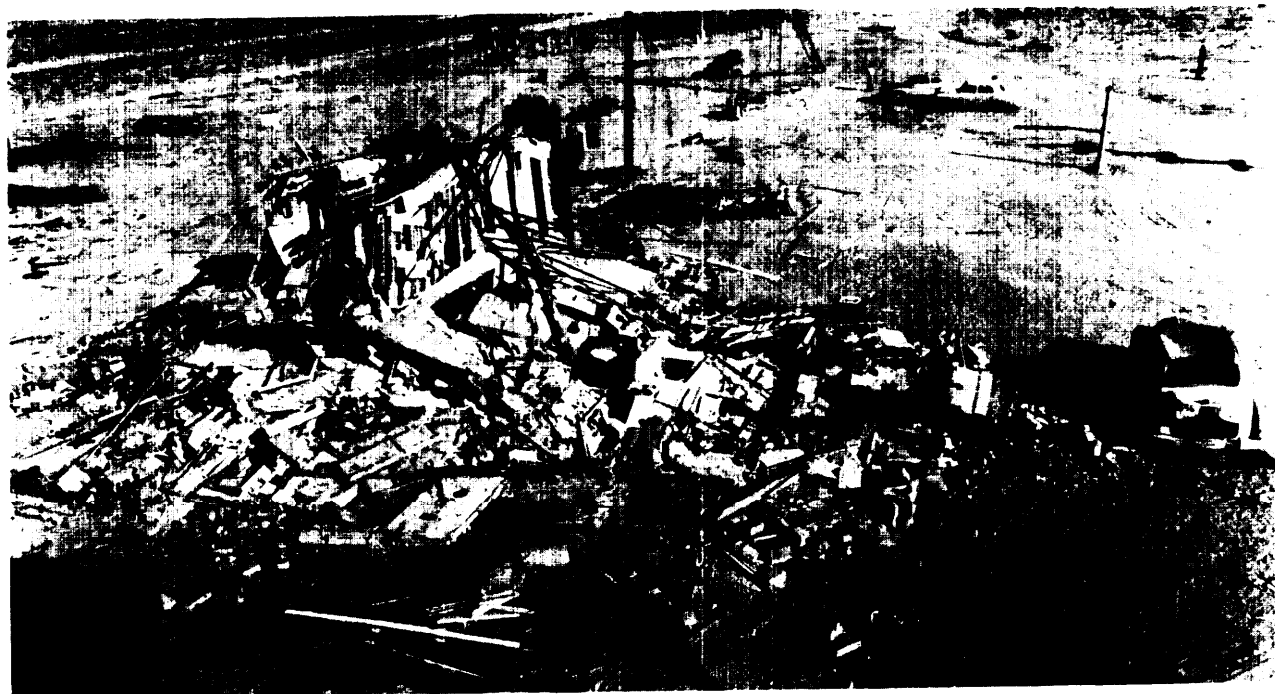
Damage to unreinforced brick house (5-psi overpressure)
